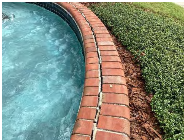
Grout and masonry deterioration
