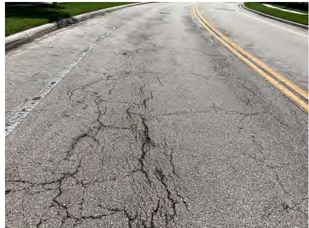
Pavement cracks at Ancient Oaks
