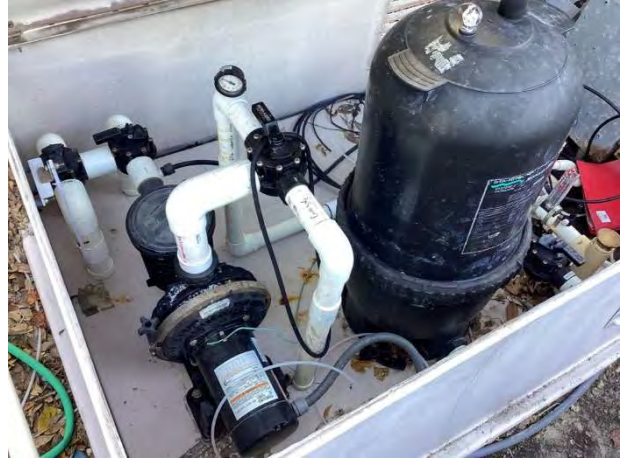
Pool pumps and filters
