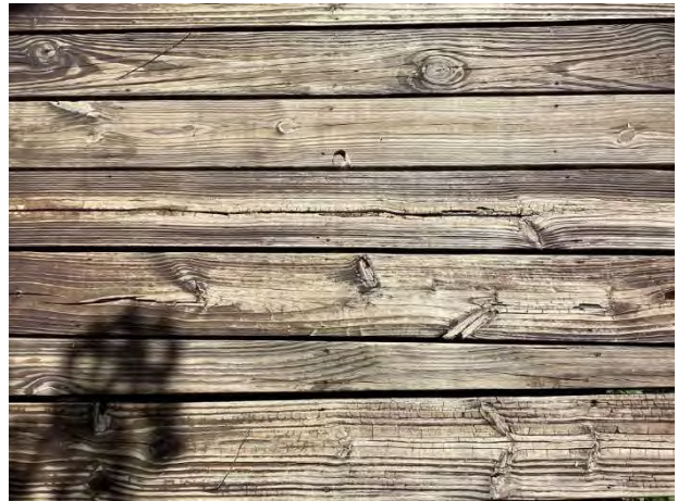
Weathered deck boards
