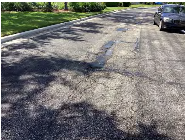
Pavement cracks and deterioration at Edenfield
