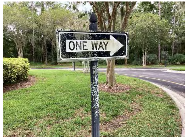
Sign finish deterioration
