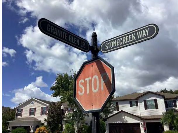
Sign finish deterioration
