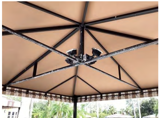
Minor frame finish deterioration
