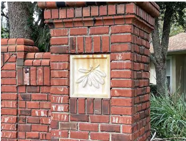
Finish stains and grout deterioration
