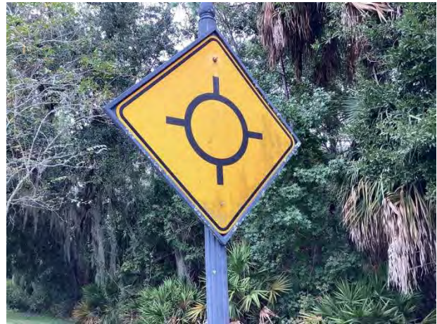
Sign finish deterioration
