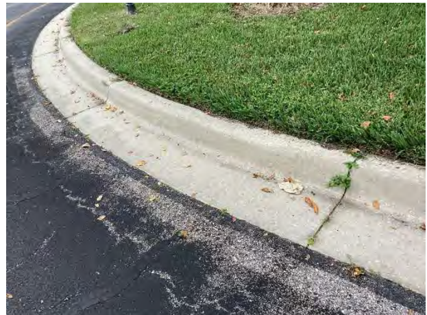
Concrete curb and gutter
