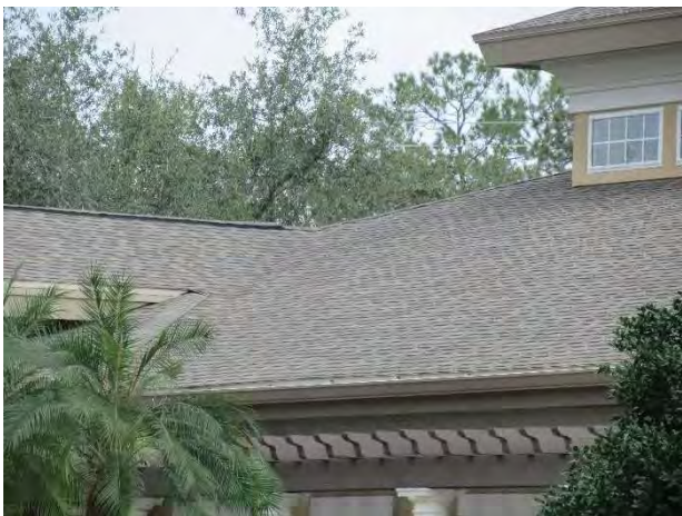
Typical asphalt shingles
