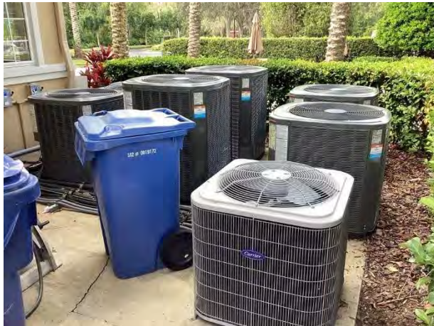
Split system condensing units
