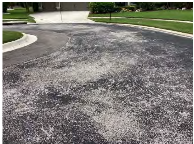
Seal coat deterioration at Forest Edge
