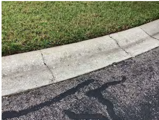
Concrete cracks
