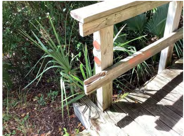
Damage at wood railing
