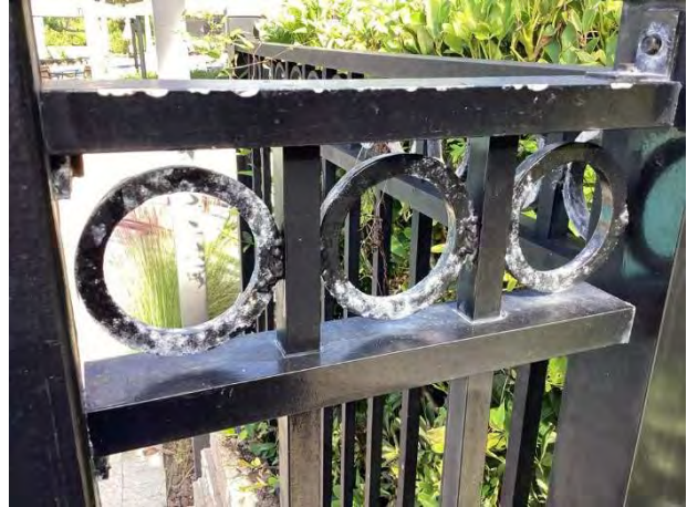
Fence finish deterioration
