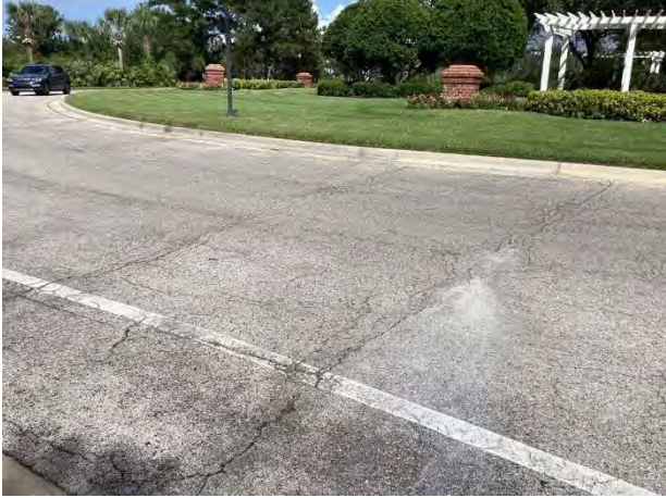
Pavement cracks at Ancient Oaks Roundabout
