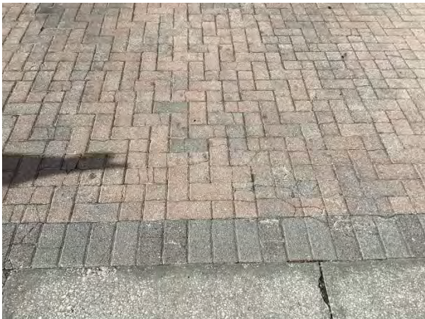
Paver cracks
