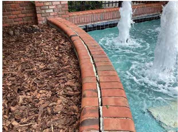
Grout and masonry deterioration
