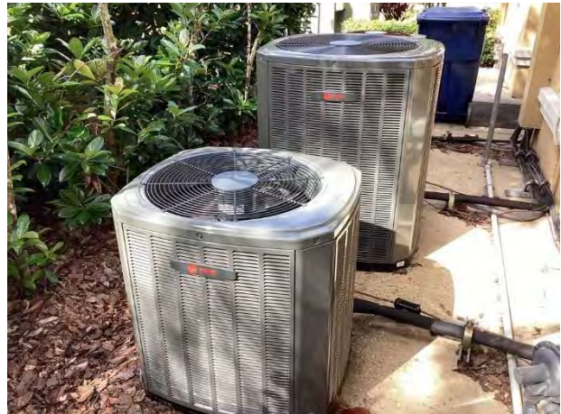
Split system condensing units
