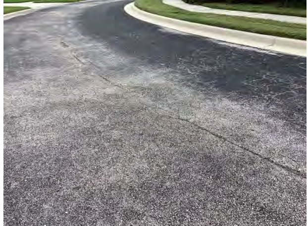
Pavement cracks at Shoregrass
