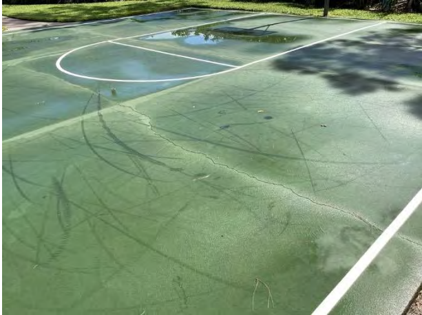
Surface cracks at Edenfield
