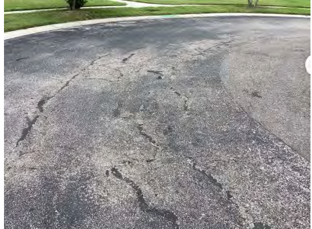
Pavement cracks at Pinecrest
