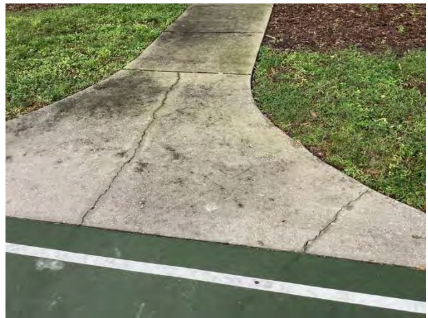
Sidewalk cracks
