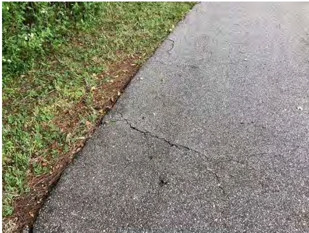
Walking path cracks
