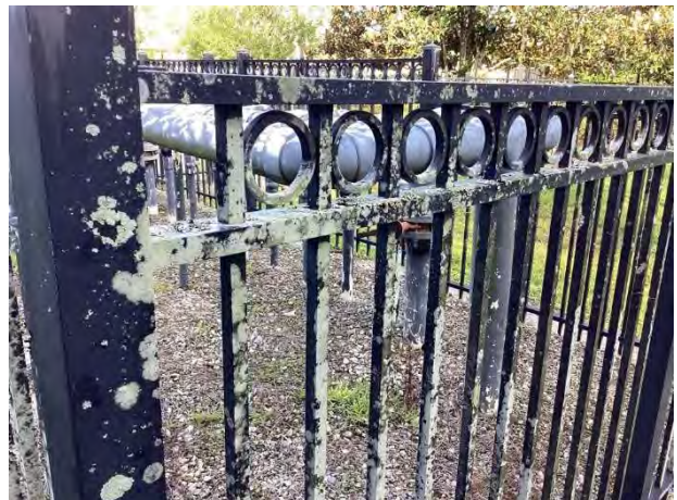
Fence finish deterioration
