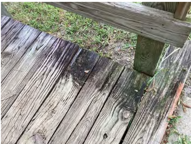
Weathered deck boards
