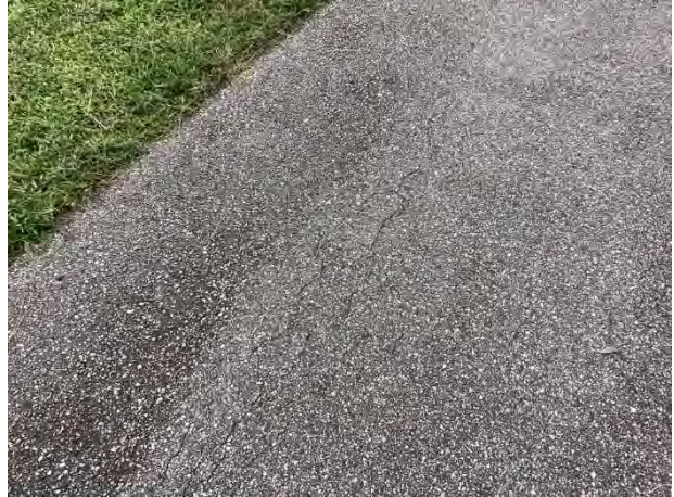
Walking path cracks
