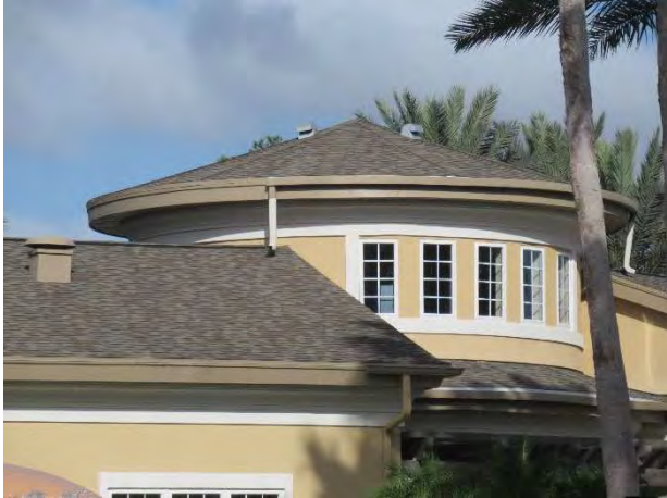
Asphalt shingle roofs at clubhouse
