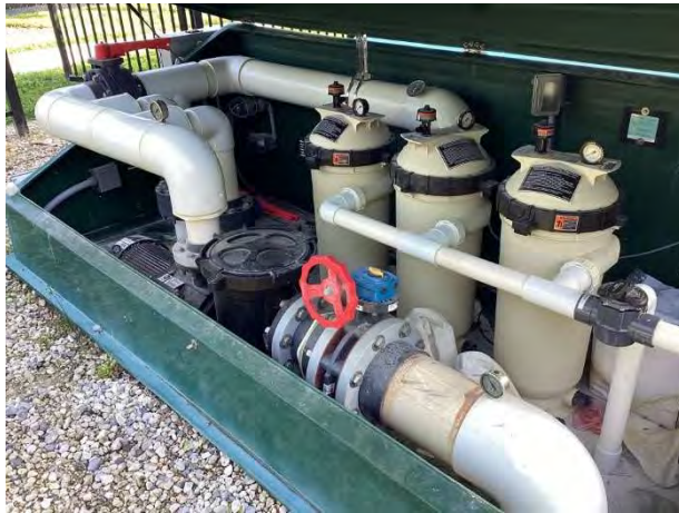
Pool pumps and filters
