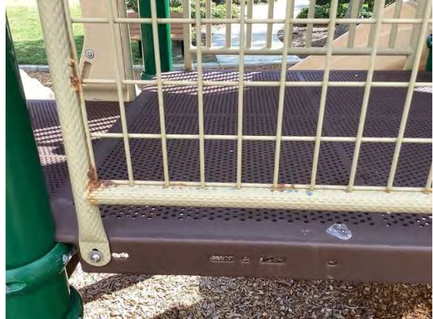
Equipment finish deterioration at Sabal Point
