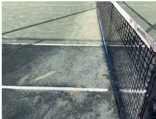
Areas of worn through clay surface
