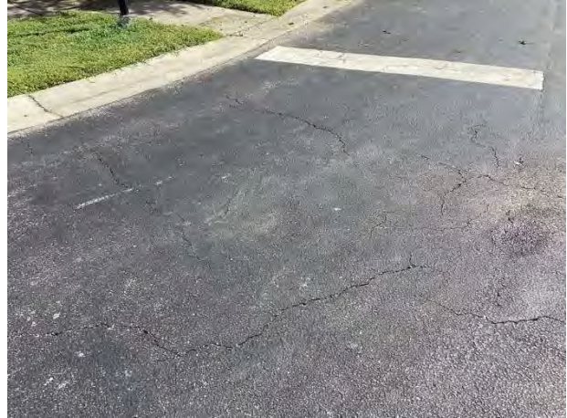
Pavement cracks at Stonecreek
