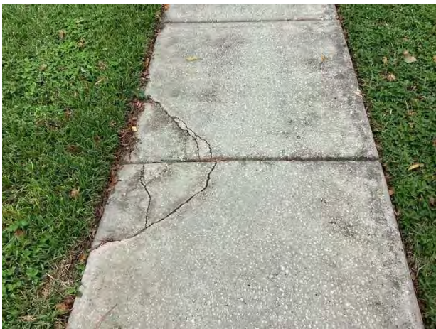
Sidewalk cracks
