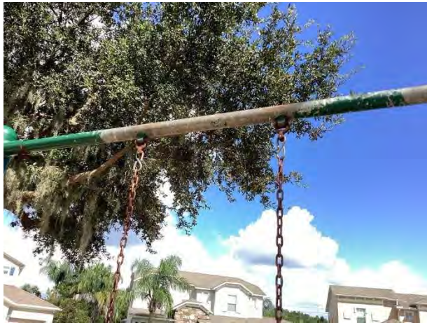
Equipment finish deterioration at Sabal Point
