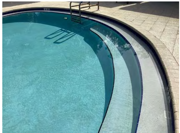
Pool plaster finish with tile perimeter
