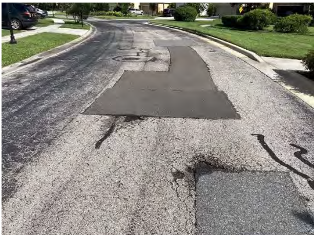
Extensive patches at Stillbrook
