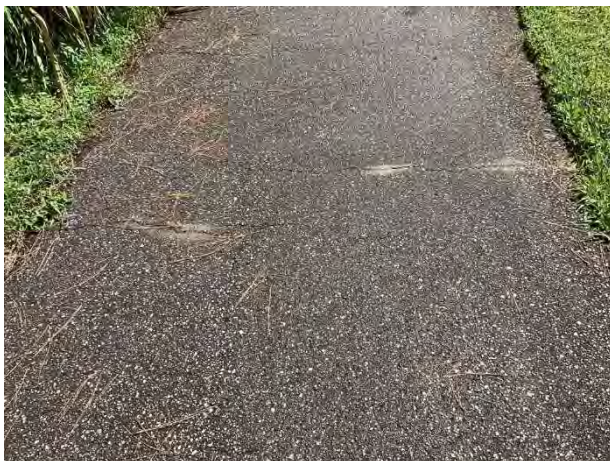
Walking path cracks
