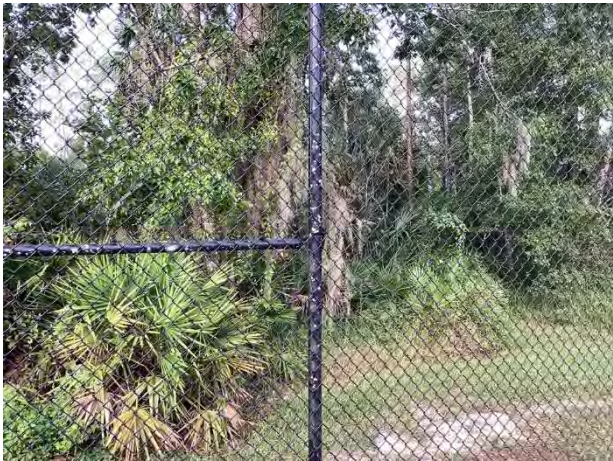
Fence finish deterioration
