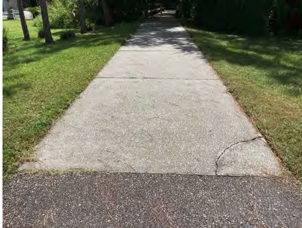
Walking path cracks
