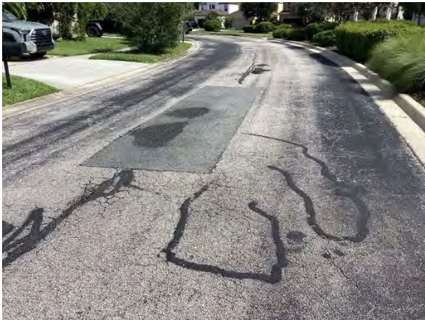
Pavement cracks and previous repairs at Stillbrook
