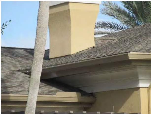
Typical gutters and metal drip edge
