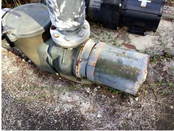
Corrosion at pump
