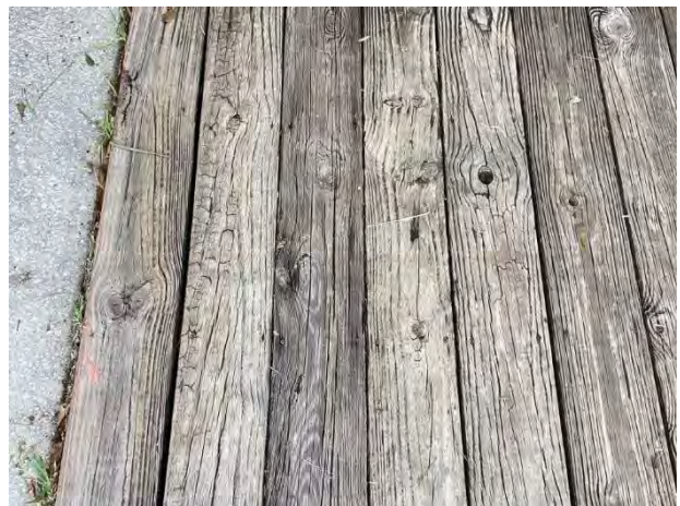
Weathered deck boards
