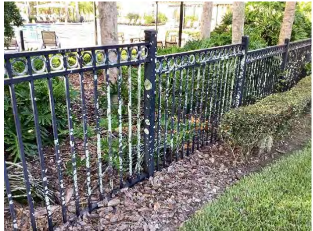
Fence finish deterioration
