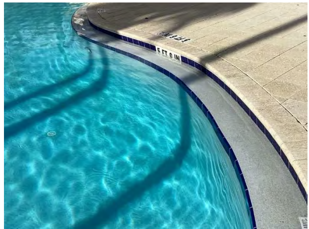
Pool plaster finish with tile perimeter
